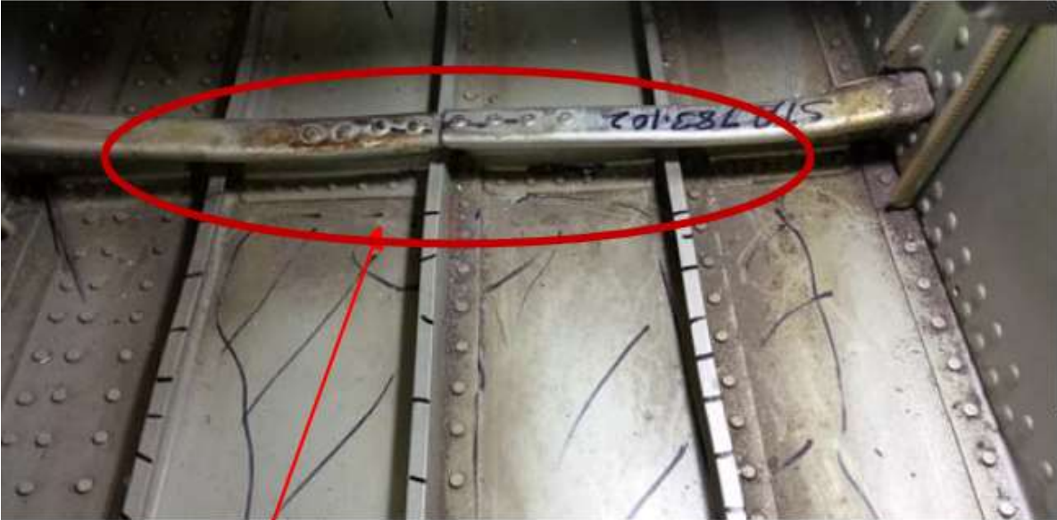
Buckling damage at Frame X783.602
