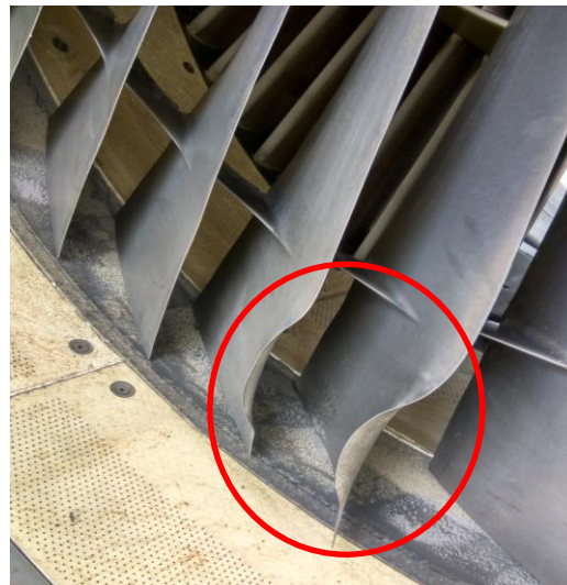
Figure # 2 Damage to Blade no. 21 & 22
